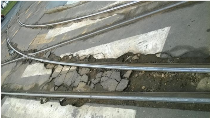
Crossing of tram track
