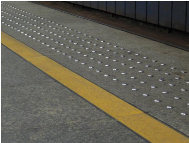
Tactile surface on the platform
